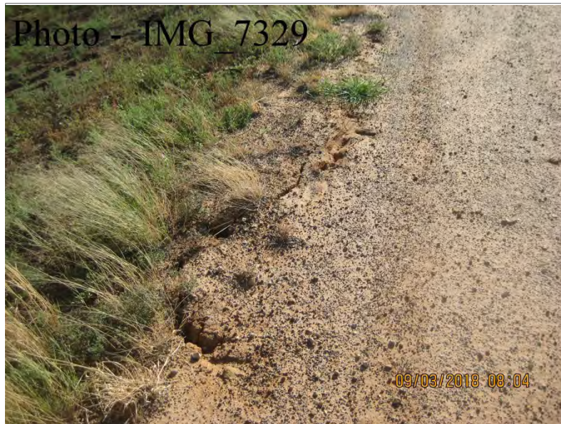
Ch. 50 – Crack River Side of Crest
