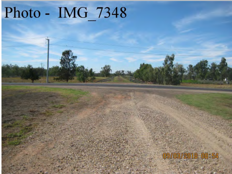
Ch. 2150 – Looking South East
