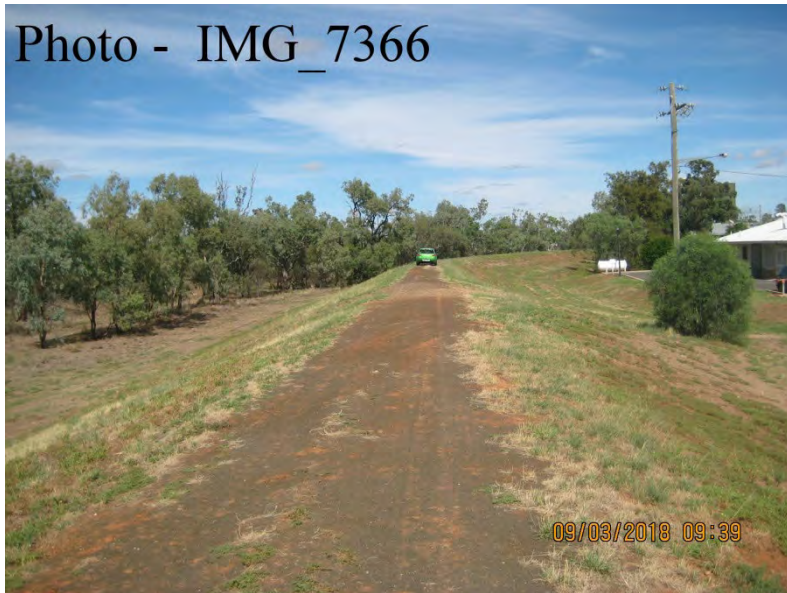
Ch. 3600 – Unformed Crossing, S End of River Rd.
