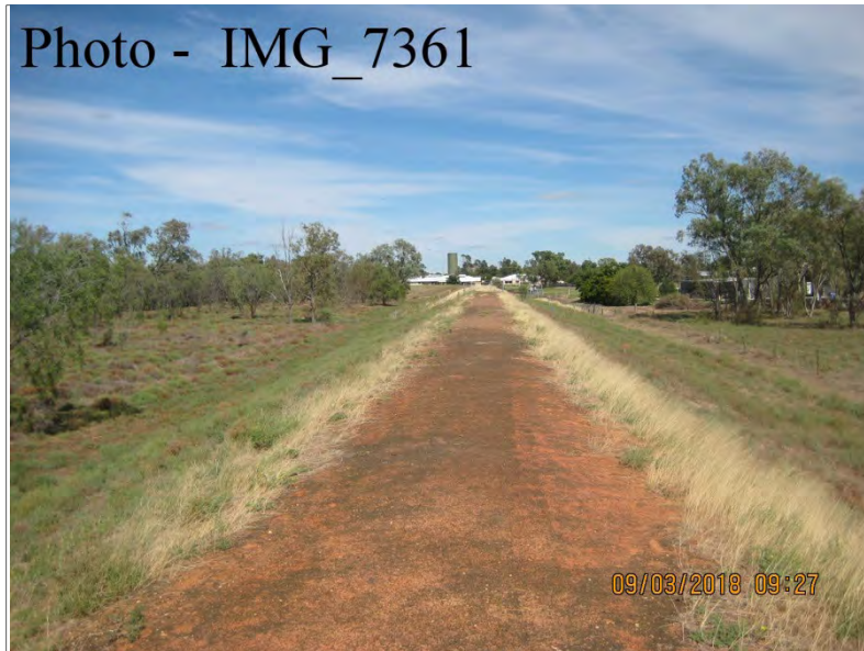
Ch. 3100 – Looking West
