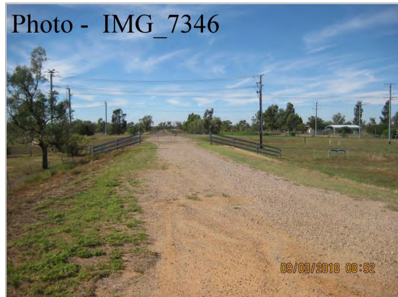
Ch 2150 – Looking South East
