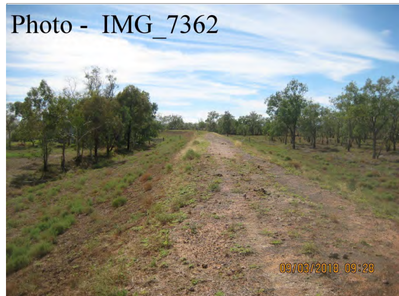
Ch 3100 – Looking East
