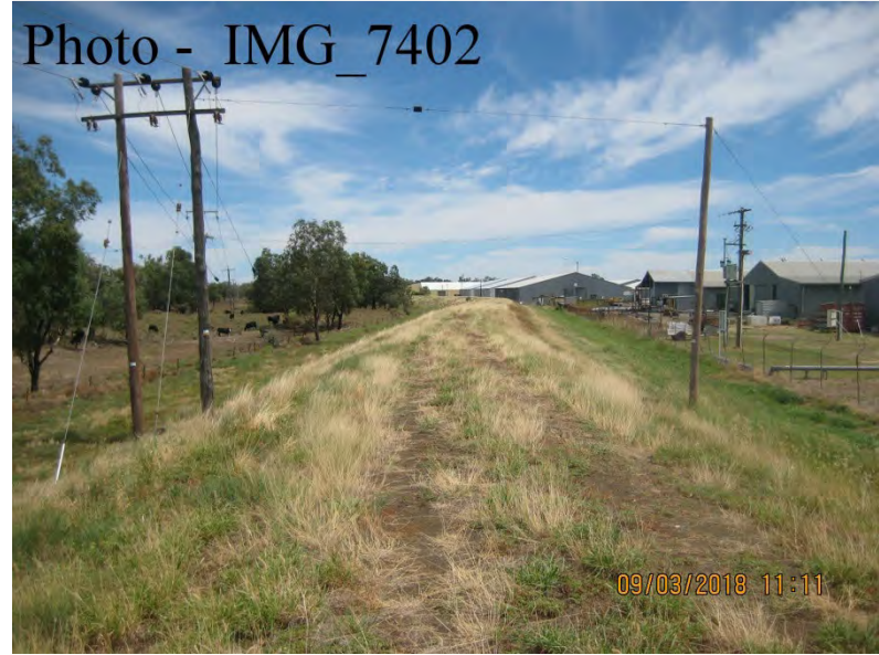
Ch 5600 – Looking West
