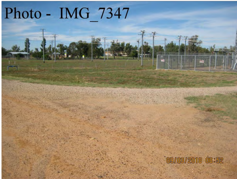
Ch. 2150– Access to Substation, Formed Crossing
