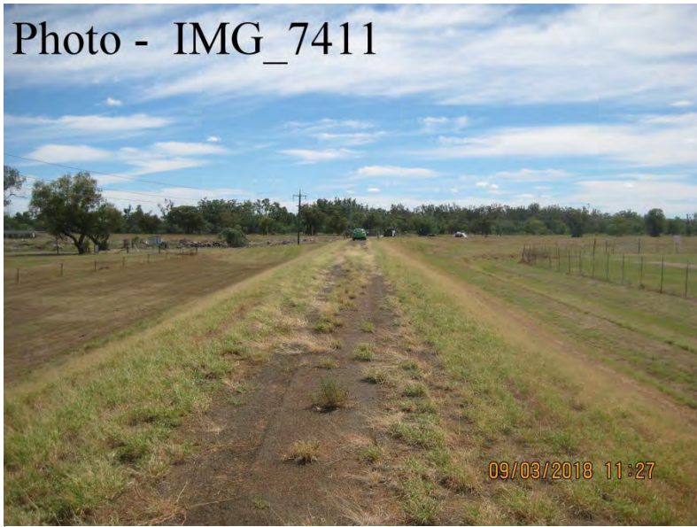
Ch. 6650 – Looking North
