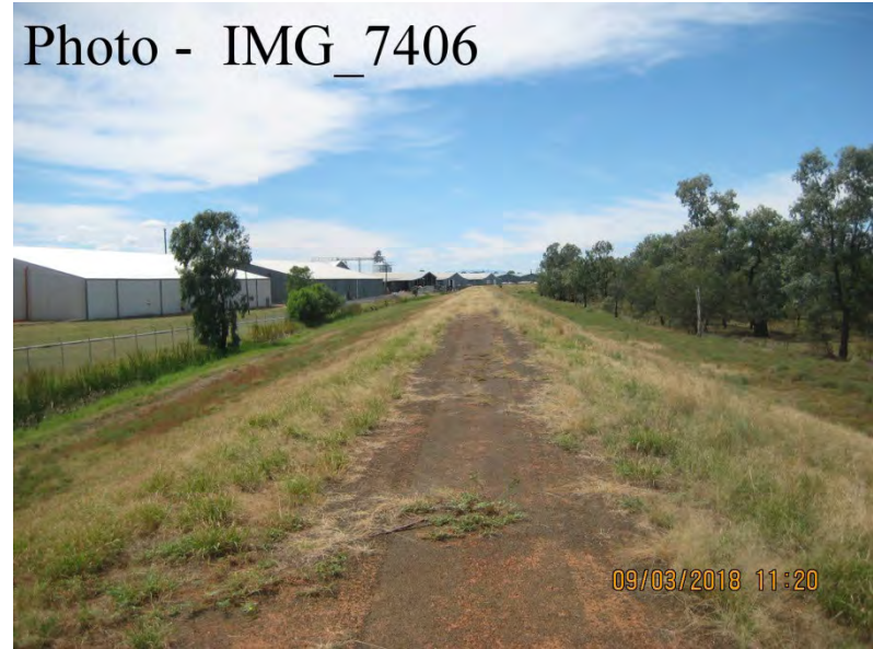
Ch 6200 – Looking East
