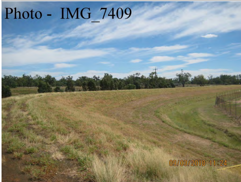
Ch. 6400 – Looking North
