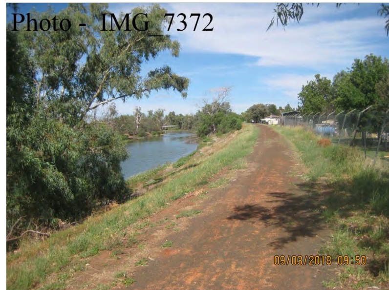
Ch 4030 – Lagoon at River Side Toe
