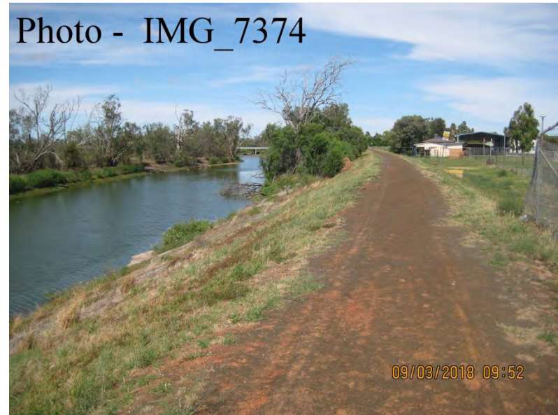
Ch 4050 – Lagoon at River Side Toe
