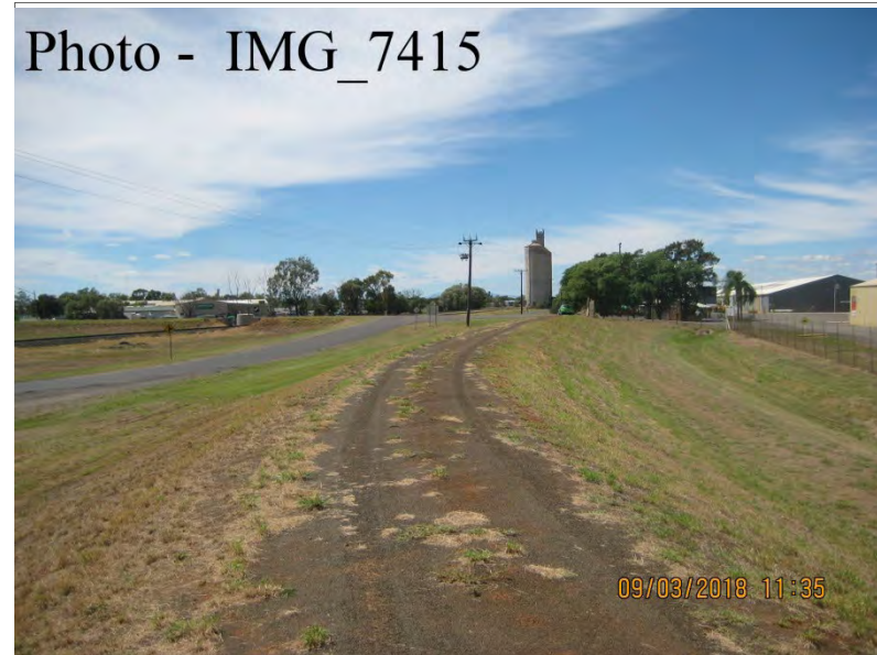
Ch 6900 – Looking East
