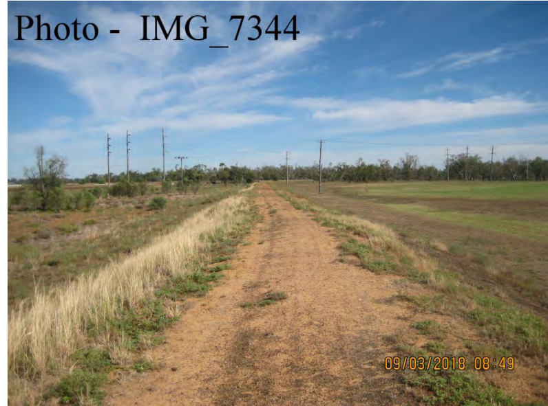
Ch 2100 – Looking North West
