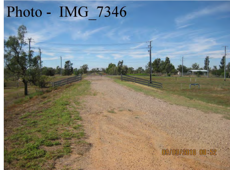
Ch 2150 – Access to Substation, Formed Crossing
