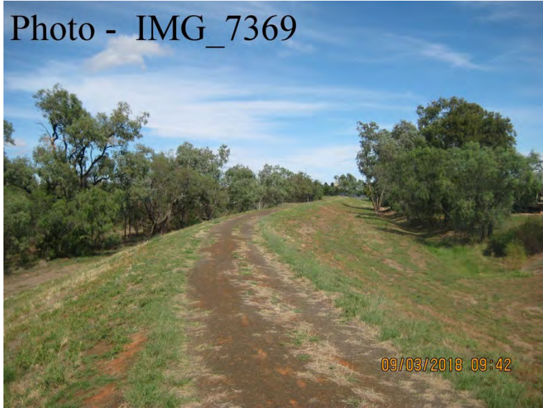
Ch. 3650 – Looking West
