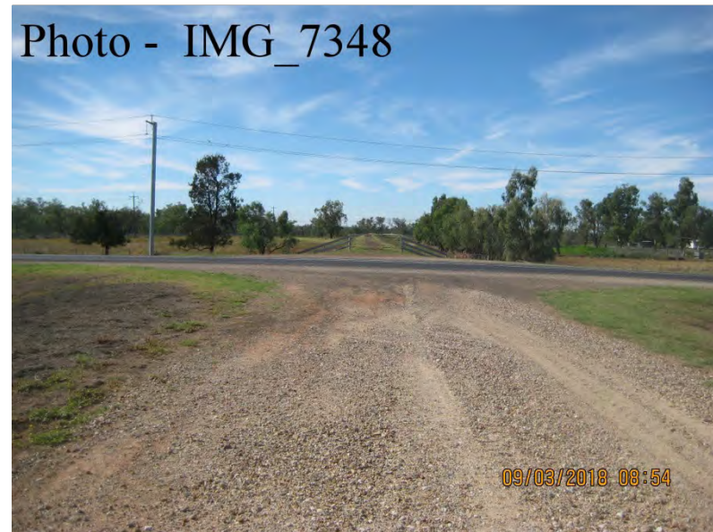
Ch 2200– Kamilaroi Highway, Sealed Crossing
