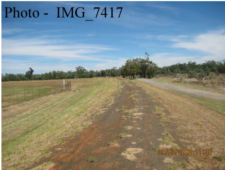
Ch. 6900 – Looking West
