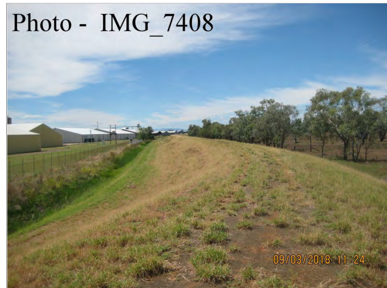
Ch 6400 – Looking East
