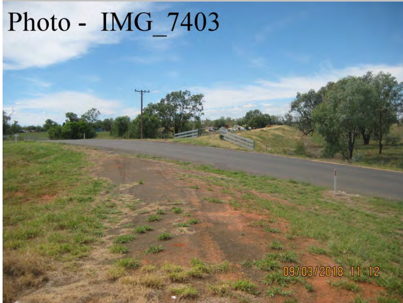
Ch. 5600 – Looking East
