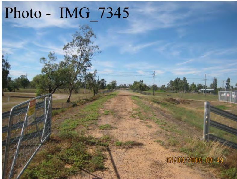
Ch 2100 – Looking South East
