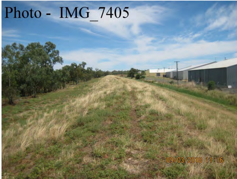
Ch. 5900 – Looking West
