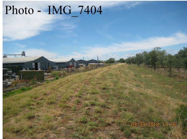
Ch 5900 – Looking East
