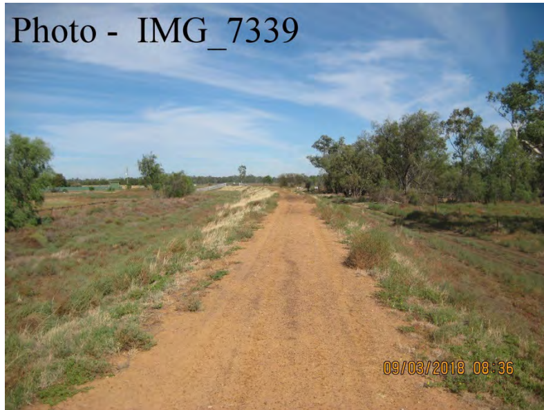
Ch. 1250 – Looking West
