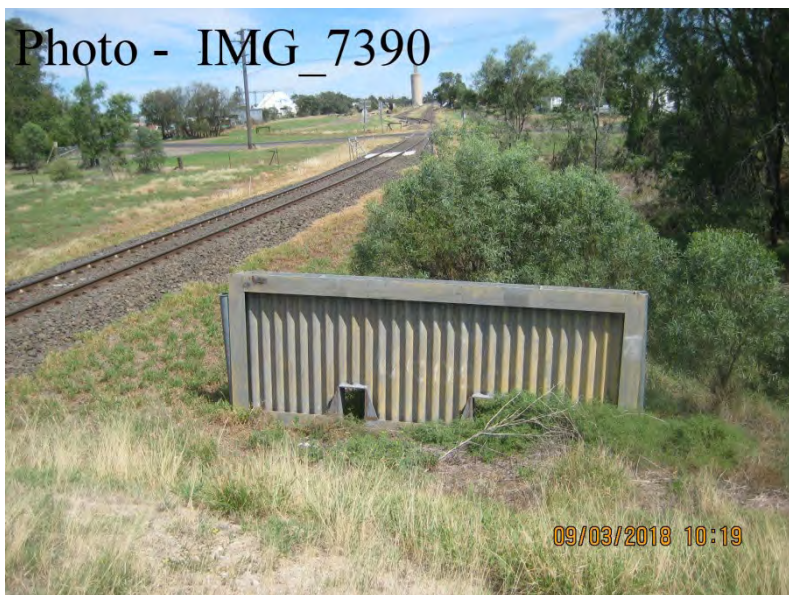
Ch. 4700– Flood Gate for Eastern Rail Crossing
