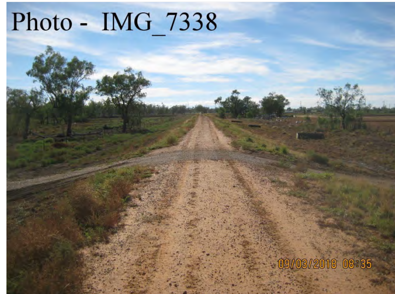
Ch 1250 – Looking East
