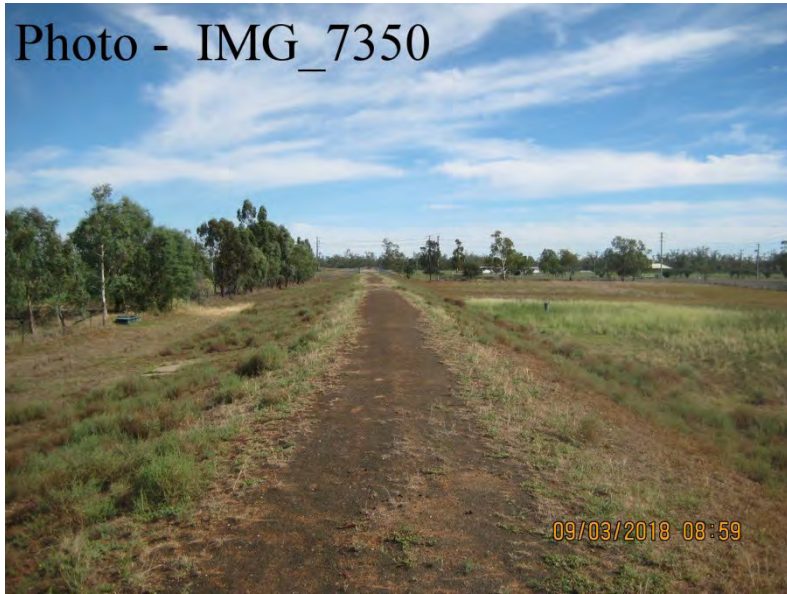
Ch. 2450 – Looking North West
