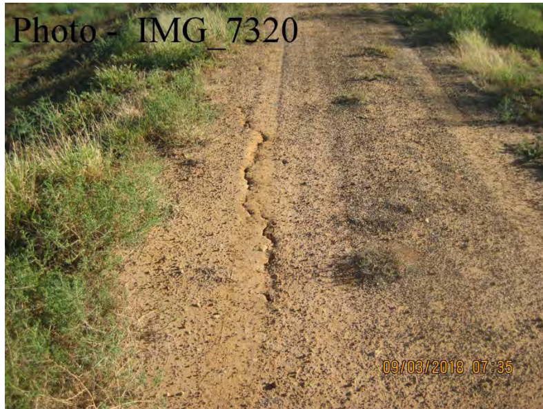
Ch. 7950 – Crack River Side of Crest
