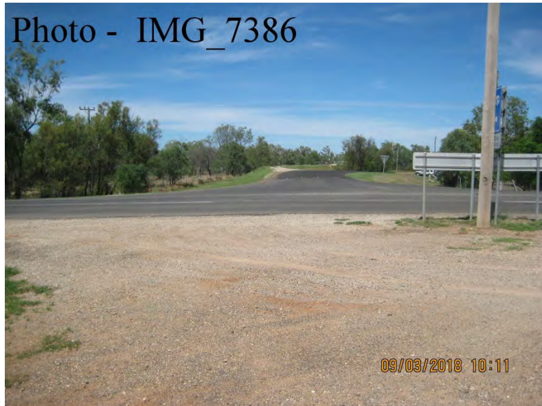
Ch. 4550 – Culgoora Road, Sealed Crossing
