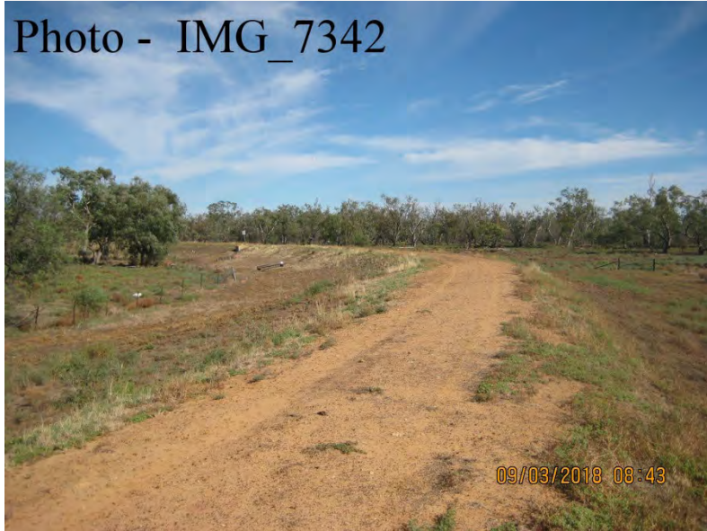
Ch. 1650 – Looking West
