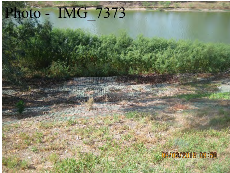
Ch. 4050 – Reno Mattress at River Side Toe
