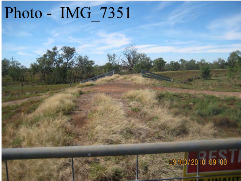
Ch. 2450 – Alama Road Unsealed Crossing
