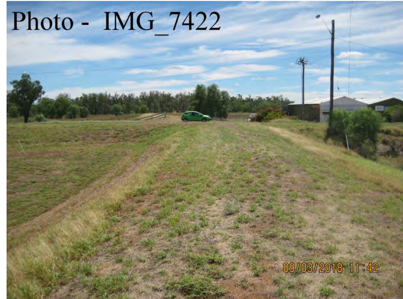
Ch 7050 – Looking North
