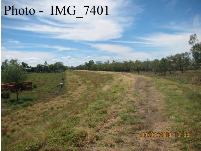
Ch. 5350 – Looking East
