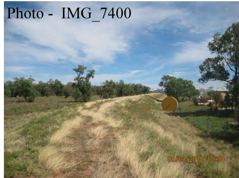
Ch 5350 – Looking North West
