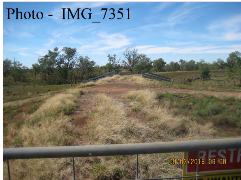
Ch 2450 – Looking South East
