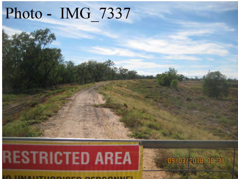
Ch. 1100 – Looking East
