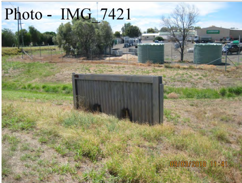
Ch. 6700 – Flood Gate for Western Rail Crossing
