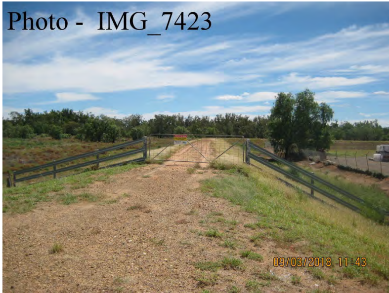
Ch. 7100 – Looking North
