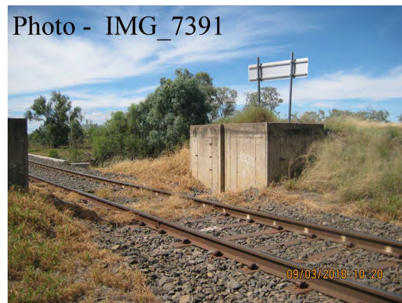
Ch 4700 –Eastern Narrabri/Walgett Rail Crossing
