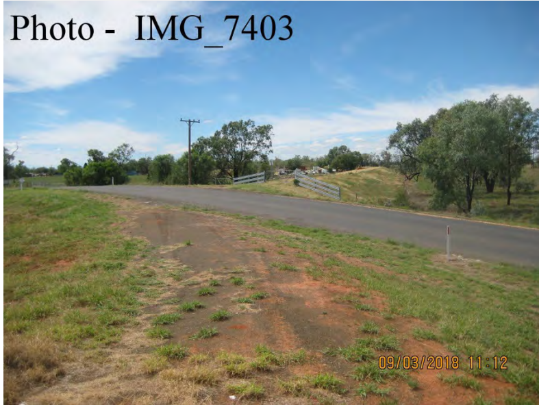
Ch. 5600 – Leap Road, Sealed Crossing
