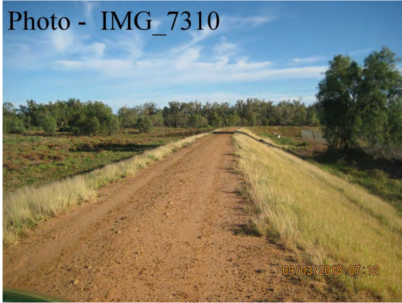
Ch. 7150 – Looking North
